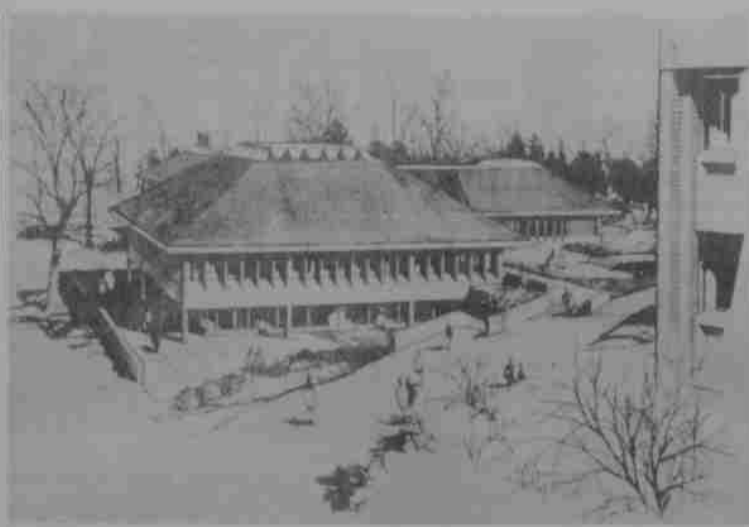
WOMEN'S DINING facilities are shown in this projection. The building is divided into three sections housing the dining area, a small reference library, and a recreation room for women.
