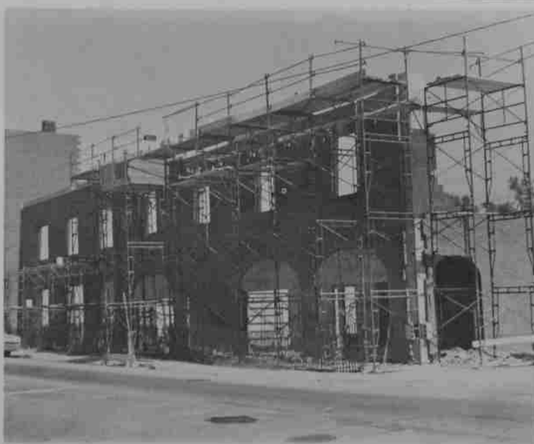
Mt. Vernon Theater in Construction
