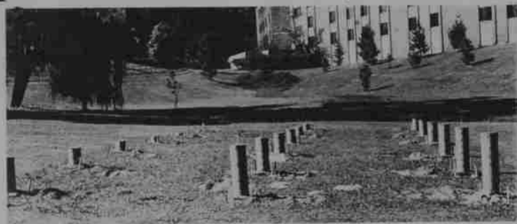
Platform tennis foundation next to Gund.
