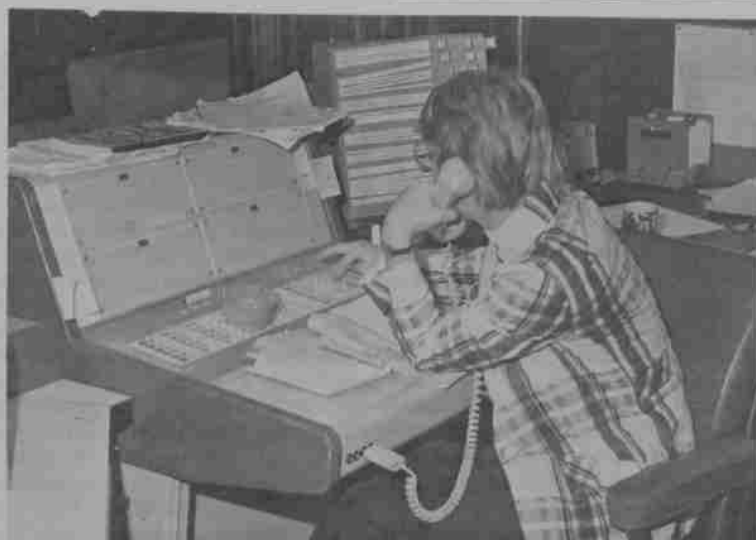
Outdated switchboard console in Ransom Hall is gone now.
