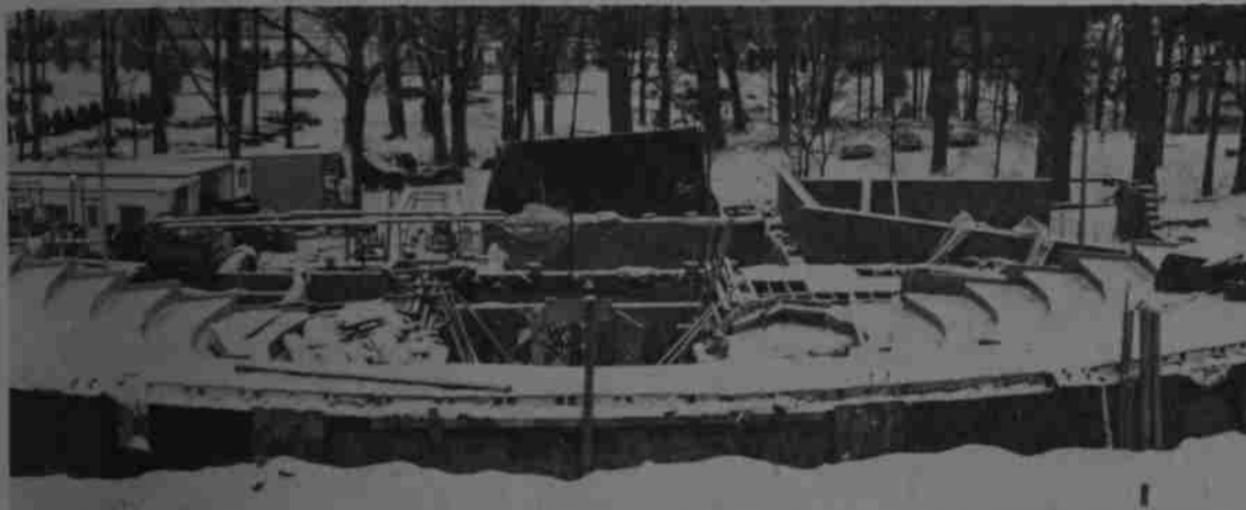
Hill Theater Under Construction
