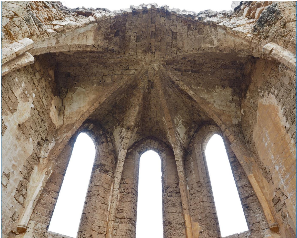
Figure 15 Famagusta, Carmelite Church, Choir Vault (vault ribs preserved only in the lower zone). Photo: author.
