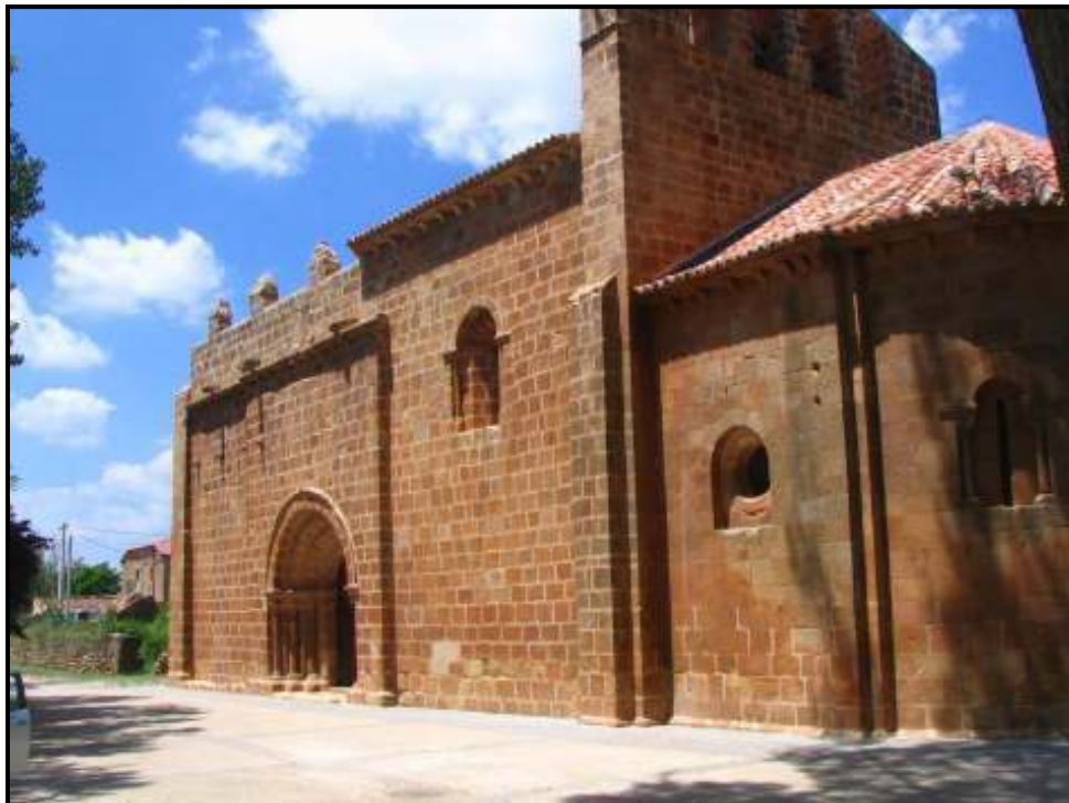
Figure 9D, Fuensauco, three building phases and fortification
