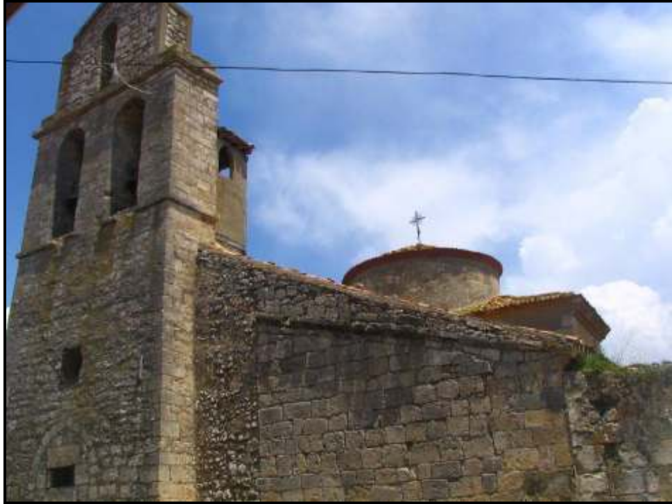
Figure 9C, Morcuera, various building materials
