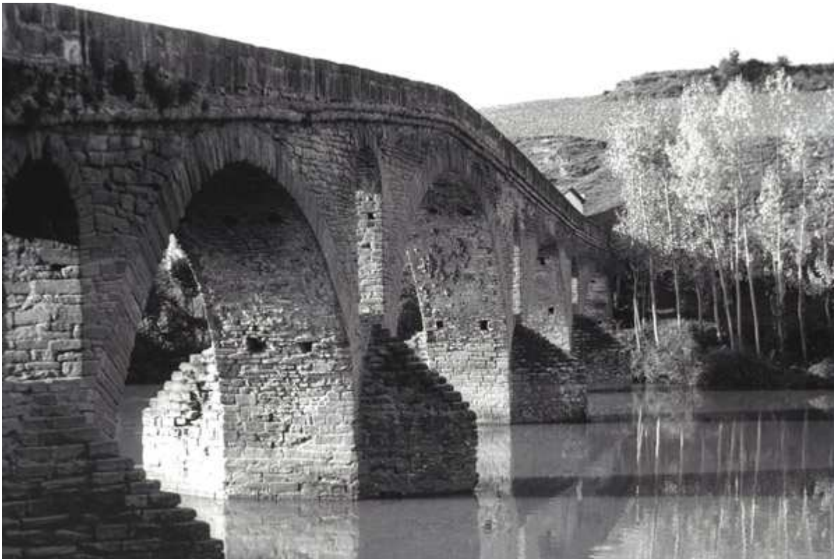
Puente la Reina Bridge Puente la Reina, Spain Photographer: W.J. Smither
